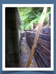
six more ties up from the pile in front of the house and began the building process. The highlight of the day--and the exhaustion of the day--was sledgehammering steel rebar into the railroad ties
